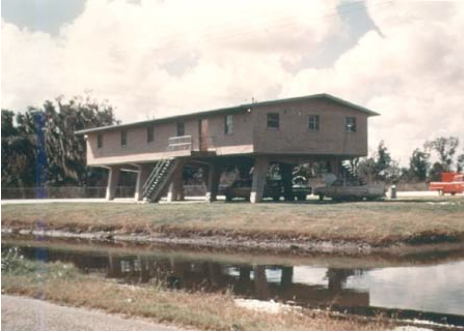
Example of a typical flood proofed structure
